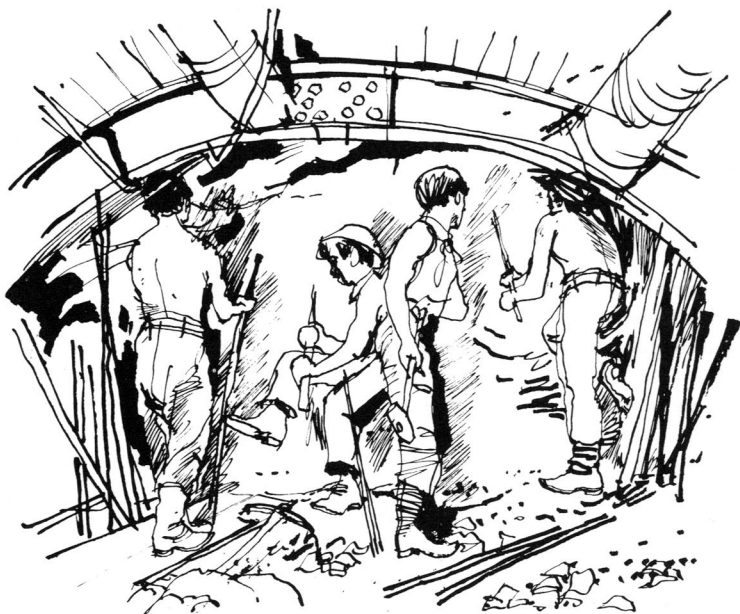
66 Men working in the Shield at the rock face in the Simplon
